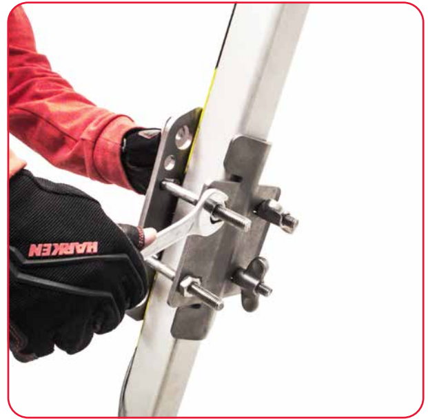
2. Tighten the two nuts with a wrench
